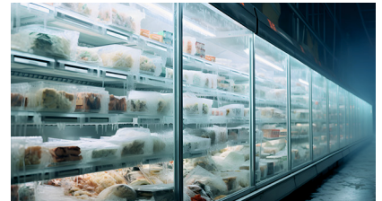
CA cold storage chambers
